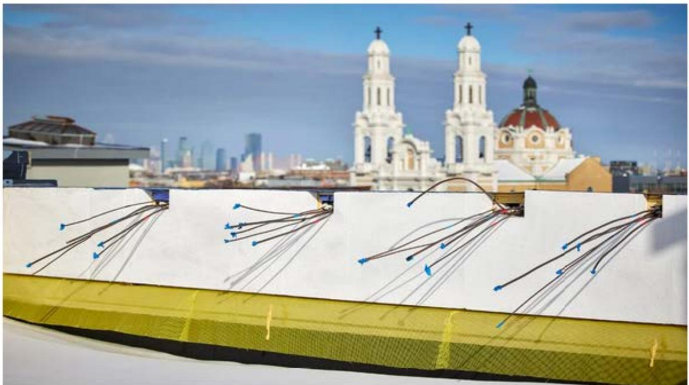
The apartments of Casa Pasiva will have heating and air-conditioning units connected to a system of ducts and refrigerant lines that snake up the walls and connect to a rooftop ventilator. John Muggenborg for The New York Times
